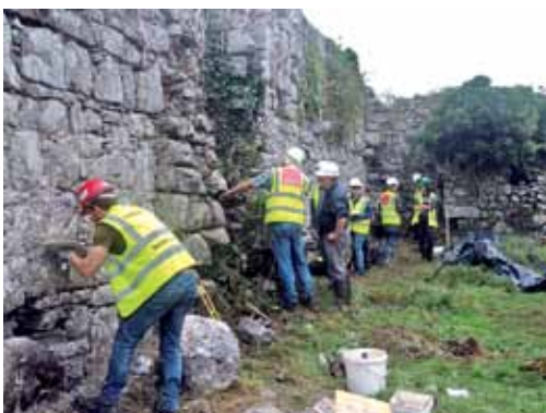
Conservation lime mortar work on the interior walls of An Cabhail Mhór.
